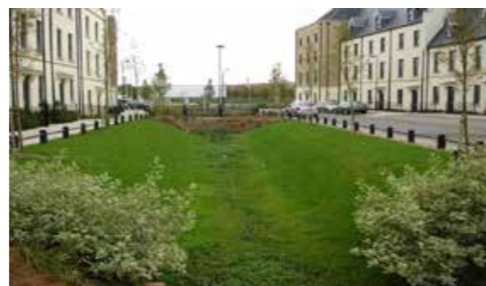
Figure 15.12 Swales at Upton, Northhampton, UK
