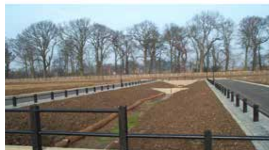
Figure 15.13 Swales at Upton, Northhampton, UK
