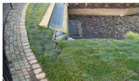
Figure 15.14 Swales at Upton, Northhampton, UK
